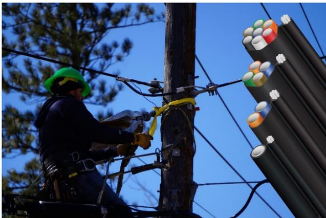
Dura-Line's FuturePath Figure-8 Aerial Self-Support is a configuration of MicroDucts with seven tubes inside the oversheath along with a
