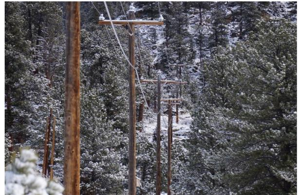
Generally, poles are placed 150 to 200 feet apart and the tension on the line is between 1,500 and 2,500 pounds. The conduit has been tested to support up to 6,500 lbs. of linear tension. This includes accounting for rain, wind, and ice loading as well as a certain amount of sag between poles.
